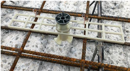
Application on bottom plates or slabs, the UNI-concrete sleeve will be fixed with the fitting plate to the upper reinforcing-rods.
